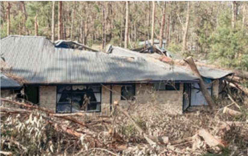
The roof caved in at this property due to the supercell storm. Ob13_1024
