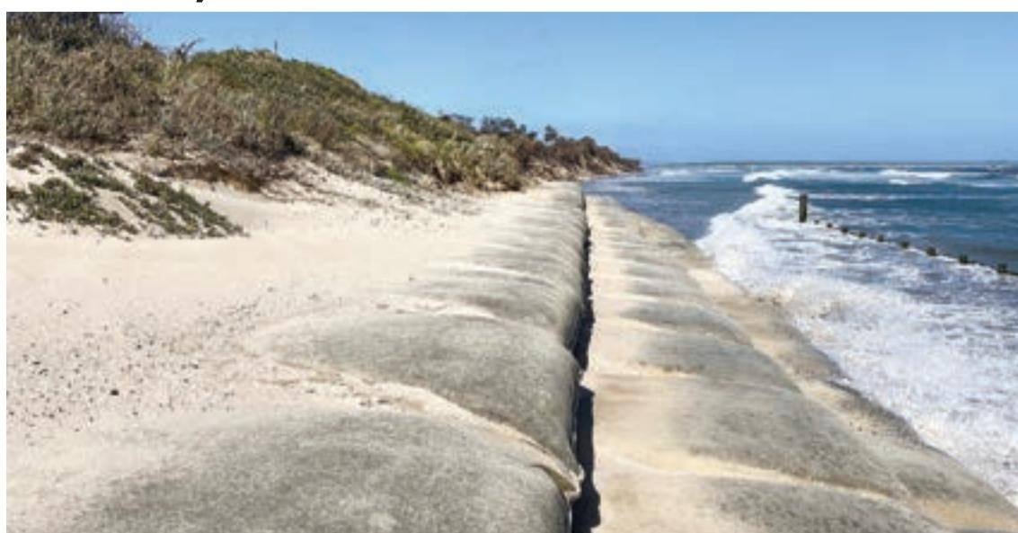
Constant pounding by the sea has reduced the effectiveness of the geotextile bag wall in front of the Inverloch Surf Lifesaving Club, while eroding the dunes at each end of the wall. The concern is that if king tides through April combine with storm surges, it could spell catastrophe for the surf club.
