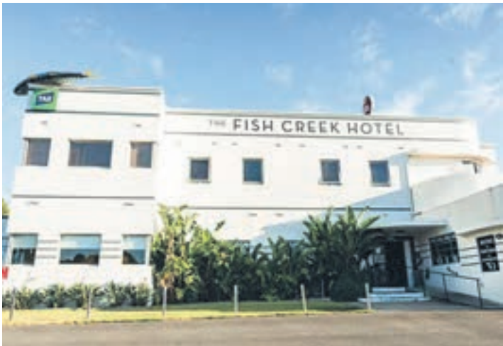
Built in 1939 in an Art Moderne style, is the iconic Fish Creek Hotel, which currently has no heritage overlay to protect it, like many other places of significance across South Gippsland.
