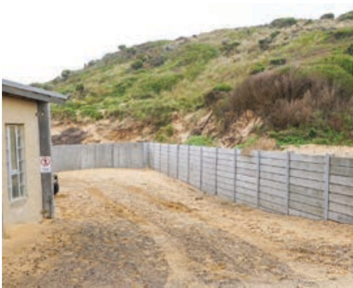
The retaining walls are proving essential to improving access to the club and stabilisation of the dunes.
