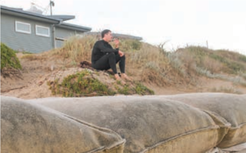
Matthew McGannon looks over sand erosion damage at the Inverloch SLSC. B21_2525
