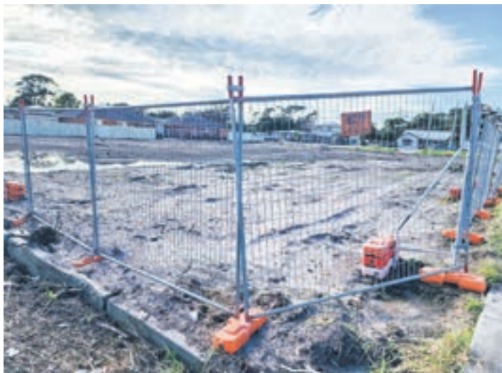
The future site of a proposed service station on the corner of McKenzie Street and Korumburra Road after demolition.
