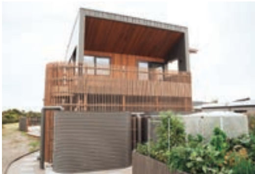
The 8.0-star home was built with 8.8kW of PV and 12kW/hr of Redback batteries, and 46,000 litres of water storage.
