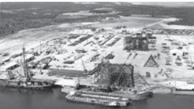
Many of our offshore platforms were originally fabricated at Barry Beach Marine terminal in the '60s, '70s, and '80s
