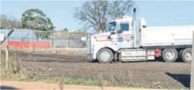
A bogged truck may have led to the collapse of the roof tunnel.
