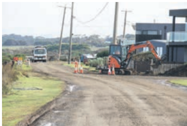
Capital works by Westernport Water are already in progress on The Esplanade at Sunderland Bay with a Special Charge Scheme to seal the road and improve drainage on the way.
