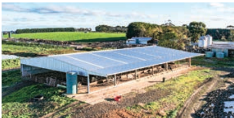
Concrete panels are manufactured in-house at Action Steel and are a recommended inclusion on a calving shed design to provide corrosion protection.
