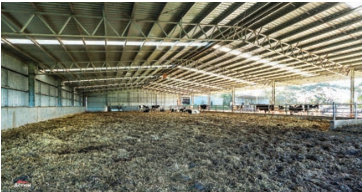
A 50m x 27m x 5m calving shed with 5 metre canopy built by Action Steel. Canopies are cost-effective additions to calving sheds for extra coverage and shelter.
