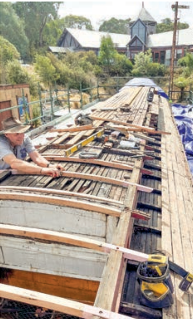
The extent of work that had to be done on train carriage restoration at Coal Creek is apparent.
