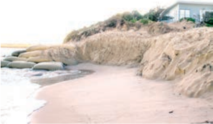
Weekend storms have taken their toll on what little sand was left to protect the Inverloch SLSC after renourishment works in June. B09_3325
