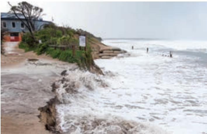
The sandbags in front of the Inverloch Surf Club are doing their work but wave action is eroding the dunes on either side of the bag wall.
