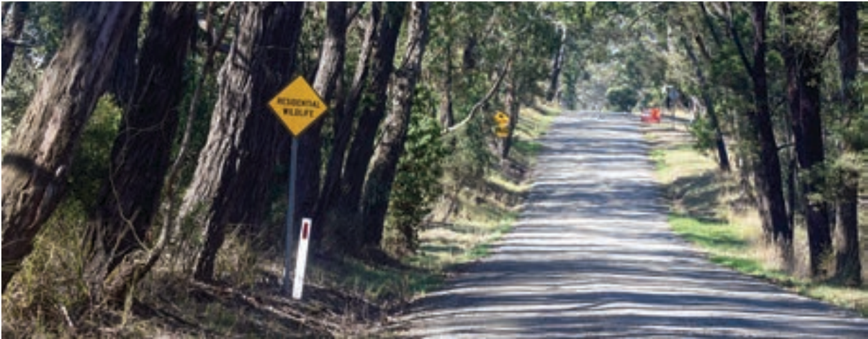
Stanley Road, a country lane, is set to become a haulage route for sand trucks.
