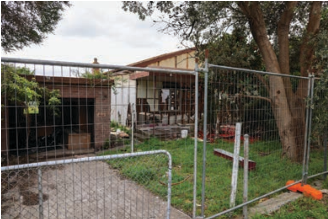
The stripped frame of 46 Hagelthorn Street, after the roof and walls were removed to deter squatters. W01_4025
