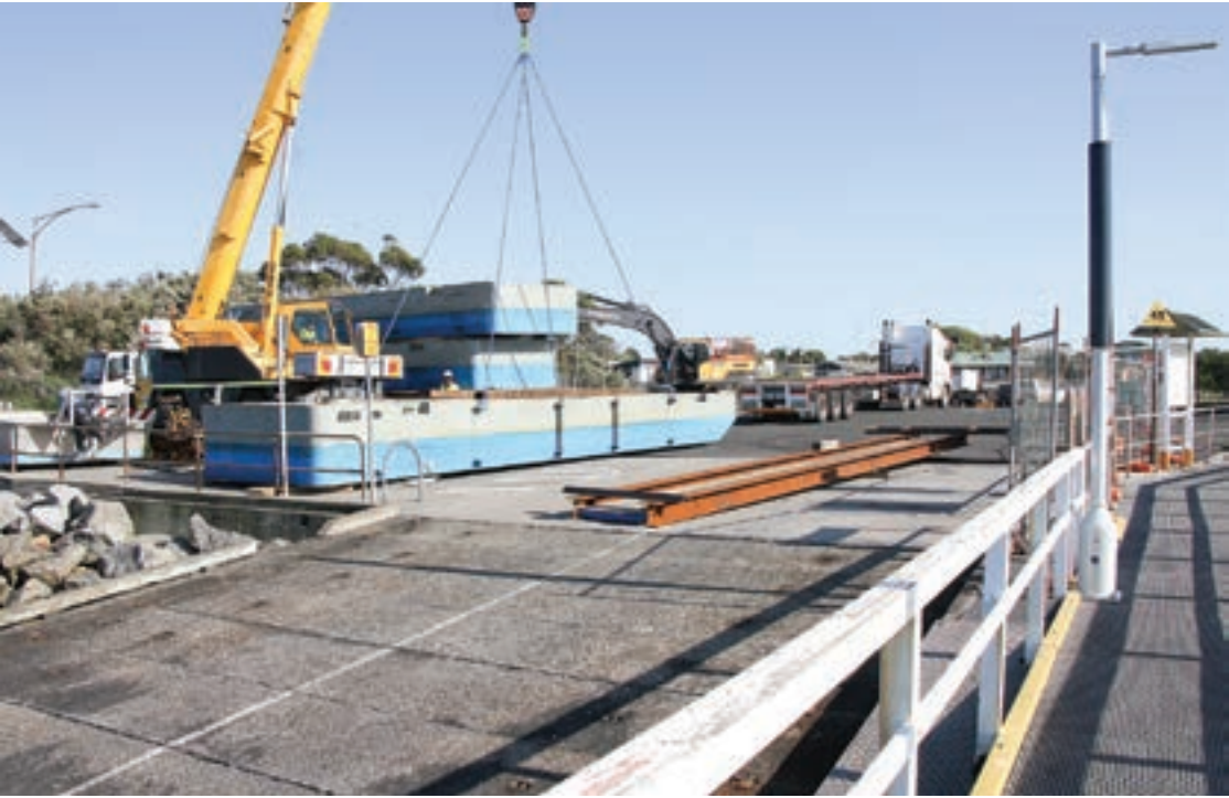
Pre-cast concrete ramps and energy-efficient lighting craned into place at the Inverloch boat ramp and jetty. B22_4124
