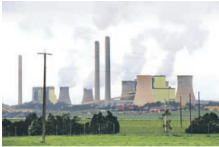
The announcement by AGL late last month of the early closure of the Loy Yang A power station, by 2023, has injected a sense of urgency into the rollout of offshore turbines along the Gippsland coast.
