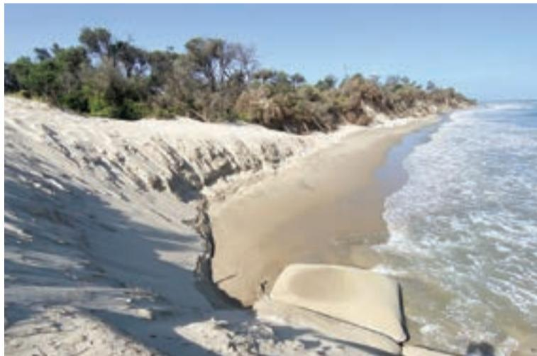
Replacing the sand on either side of the textile barrier at the front of the Inverloch Surf Lifesaving Club has only been modestly successful at best.
