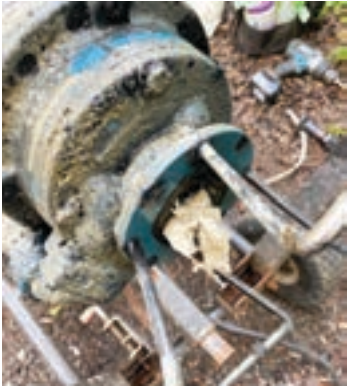
Wet wipes blocking a water pipe
