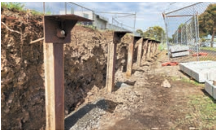
Old railway tracks were used to form the original retaining wall that is currently being rejuvenated as part of the upgrade works. C24_5023
