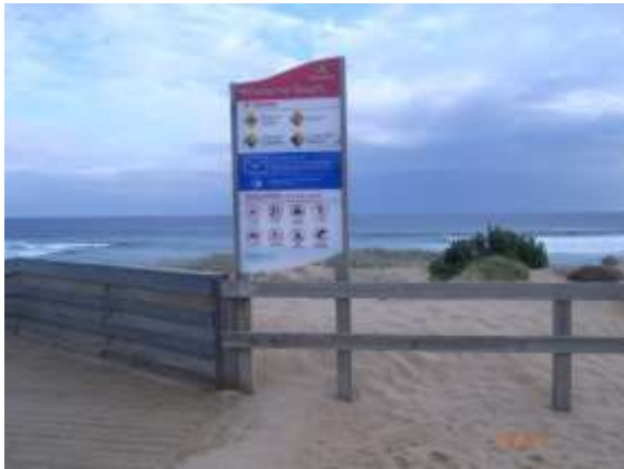
Obs 1 - Open access sign at the main beach entrance. Sign is consistent with the design intention and application clauses of AS/NZS 2416.
