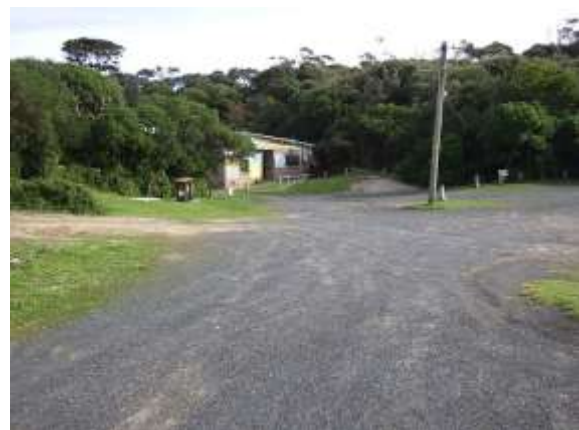
Obs 6 - View of the Wonthaggi Life Saving Club building off Bay Beach Road.
