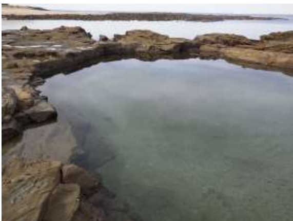
Obs 5 - View of the man-made rockpool at The Bay (Bay Beach) beach. While a good concept there are slip, trip and fall hazards associated with activity around this rockpool.
