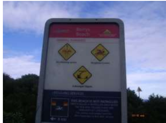
Obs 2 - Sign uses a 'No Lifesaving Service' symbol that is not found in the current AS/NZS 2416 Standard. Some water damage noted on the signs in this location.
