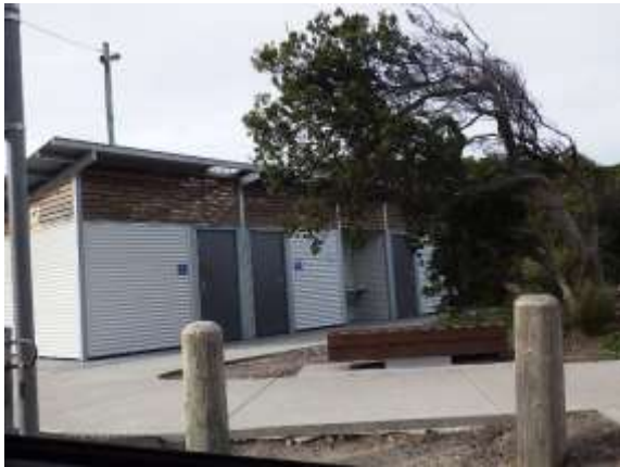
Obs 1 - Public amenities provided at Cape Paterson beach.
