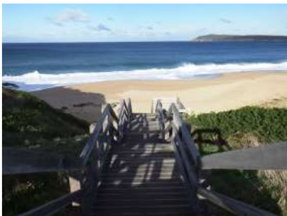
Obs 5 - Stepped boardwalk providing access to the beach.
