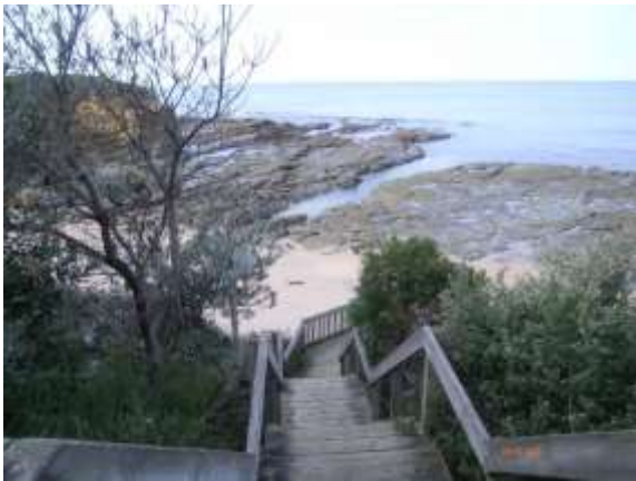
Obs 3 - Defined stepped boardwalk access provided to the beach.
