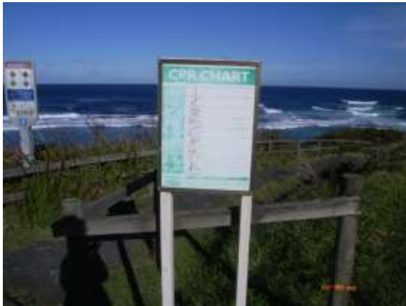
Obs 1 - A deteriorating CPR information sign noted at the top of the stairs leading down to Kilcunda West 2 beach.
