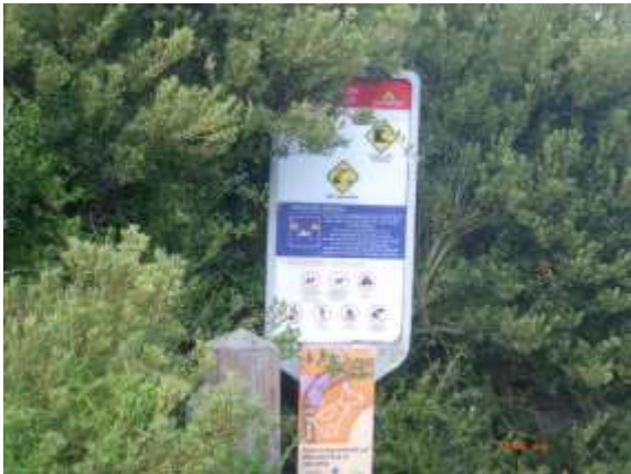
Obs 3 - Defined access sign to be repositioned of the tree foliage to be trimmed to allow an unobstructed view.
