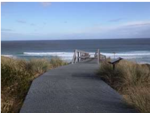
Obs 5 - Boardwalk covered with an enhanced surface to provide safer access to the beach. Interpretive signage board can be seen to the right to the boardwalk.
