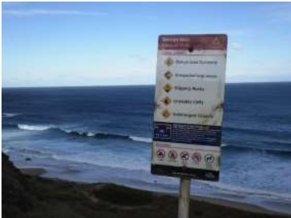
Obs 3 - Defined access sign consistent with the design intention of AS/NZS 2416. Sign placed in a location where reading it may be dangerous.
