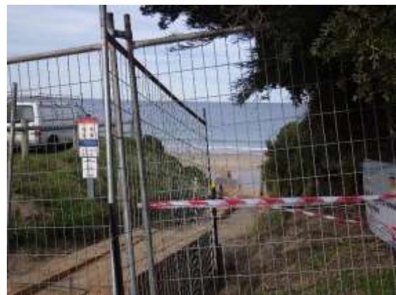
Obs 6 - Remedial works to a defined access path at the time of assessment.
