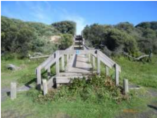
Obs 1 - Defined access path with handrail barriers down to the beach.
