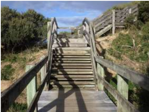
Obs 3 - Stepped boardwalk access down to the beach.
