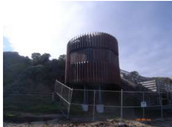
Obs 4 - View of the newly built patrol tower at Smith beach. This facility should help promote and enhance supervision services at the beach.
