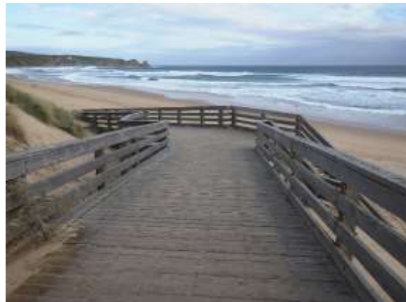
Obs 4 - Wide boardwalk access with a gentle slope providing access down to the beach.
