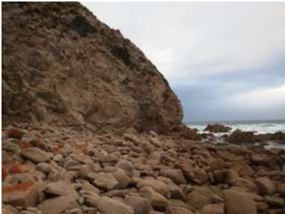
Obs 3 - Loose boulders and rocks found at the base of the headland areas.
