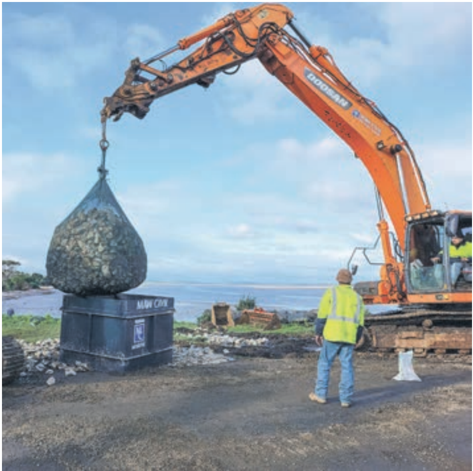
MAW Civil Marine has begun constructing a rock bag seawall at Inverloch.
