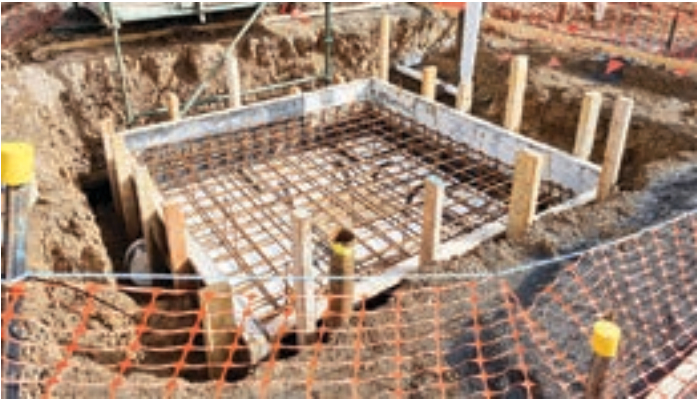
Lift pit bases being prepared for concrete.
