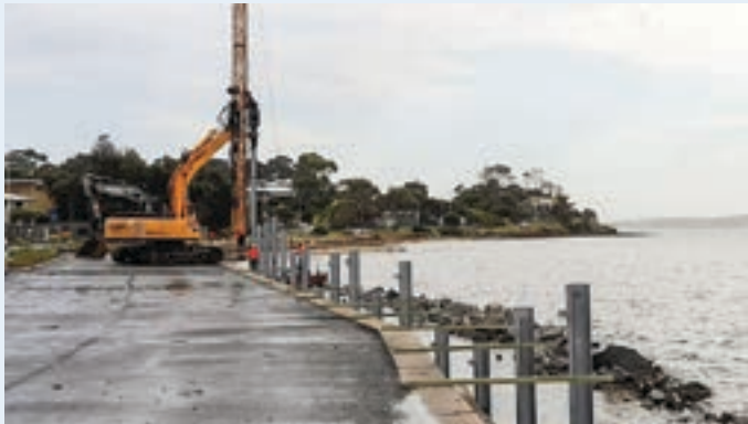
Stage 2 of the Rhyll boat ramp upgrade has seen the installation of seawall piles as well as 24 of the jetty piles.
