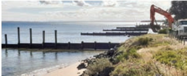
Eight timber groynes have been constructed so far at Cowes East foreshore, with the rock seawall expected to be completed by late July.
