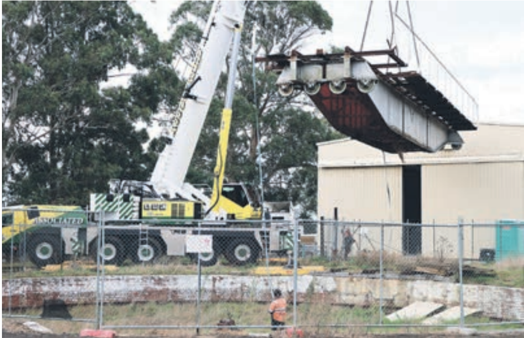
The Korumburra train turntable is removed for its trip to Yarra Glen Station. A17_2423
