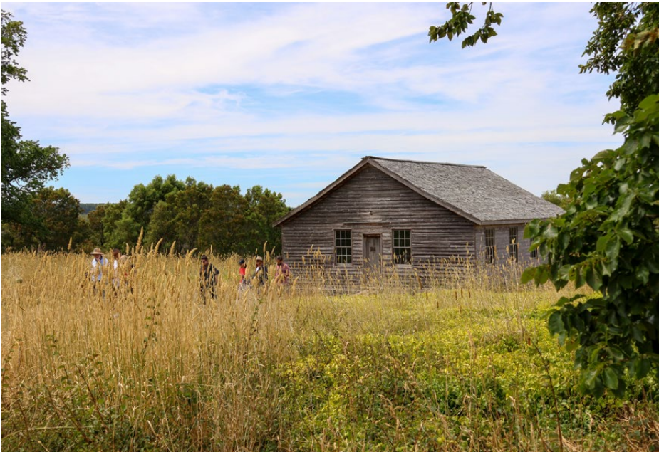
Former mission site at Lake Condah, February 2023
