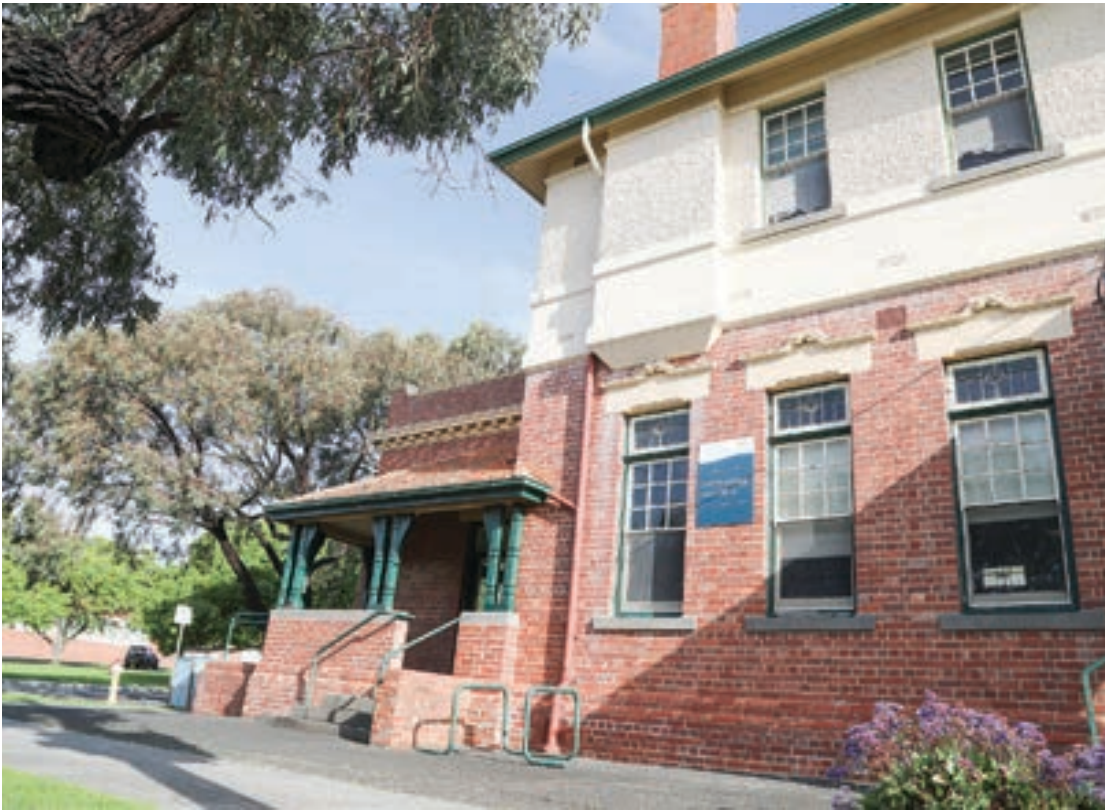
The grand old Wonthaggi Post Office is set for a $1 million internal refurbishment, making it ready for a new future, predominantly hosting community events.
