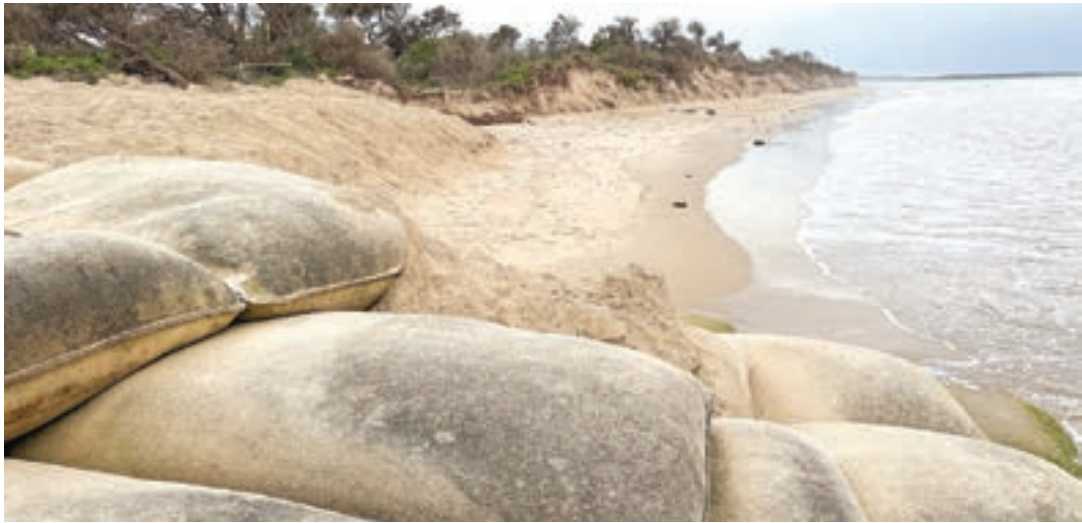
The sandbag wall in front of the Inverloch Surf Lifesaving Club will be extended east and west over the next few months, that work being completed by Christmas.
