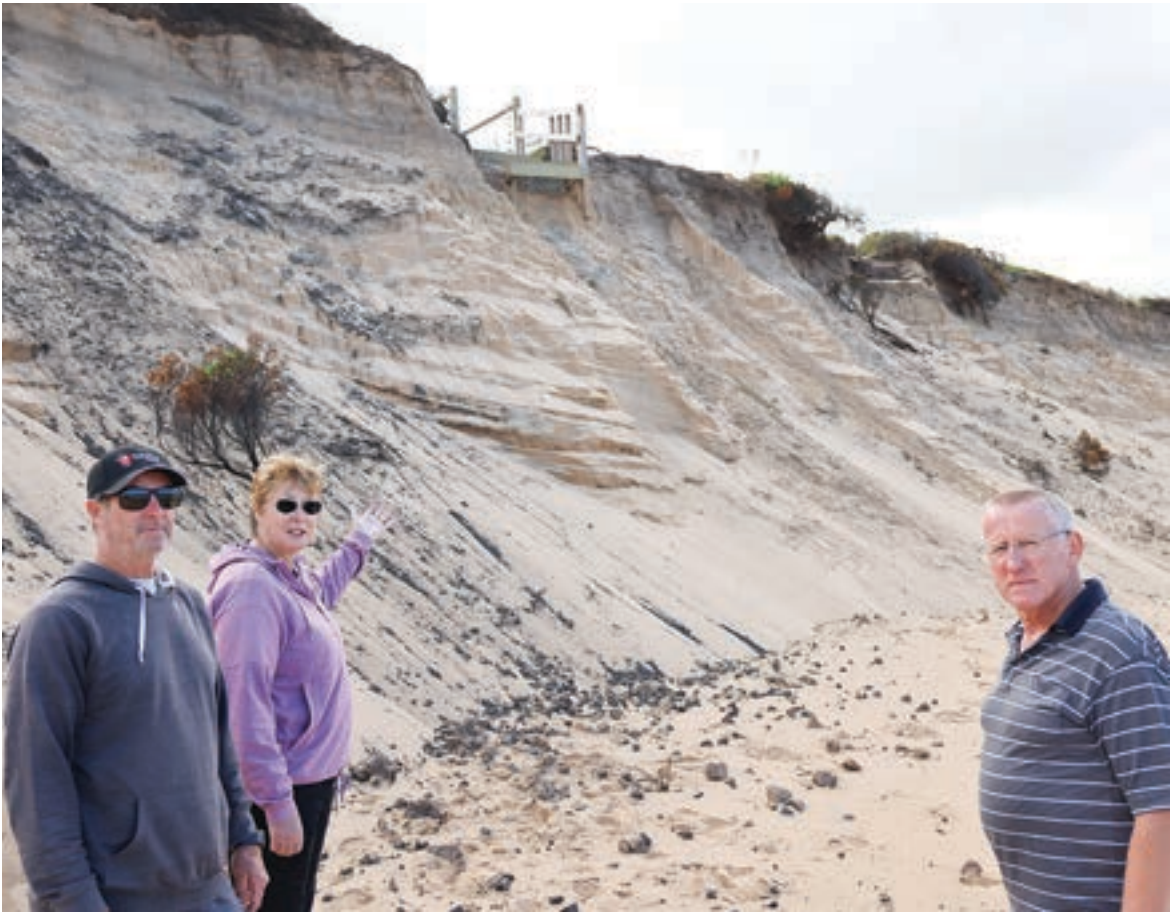
Kilcunda Community Association members Allan Richardson, Marianne Van Den Bronk and president Marcel Van Den Bronk stand beneath the collapsed staircase site at the Lionel Rose car park, where ongoing erosion threatens the rail trail above. W01_4425
